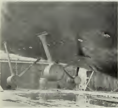
(9) Looking aft from drydock floor
